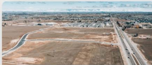
North Ranch Business Park
